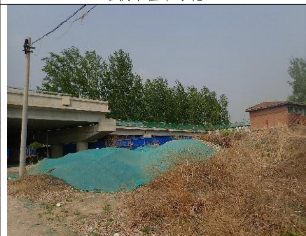
纤维网临时苫盖
