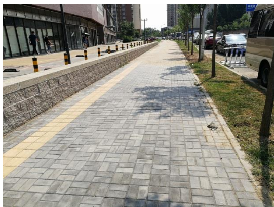
步道透水铺装及绿化带 (2020.6)
