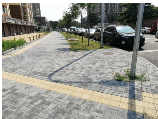
步道透水铺装及绿化带 (2020.6)
