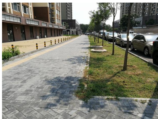
步道透水铺装及绿化带 (2020.6)
