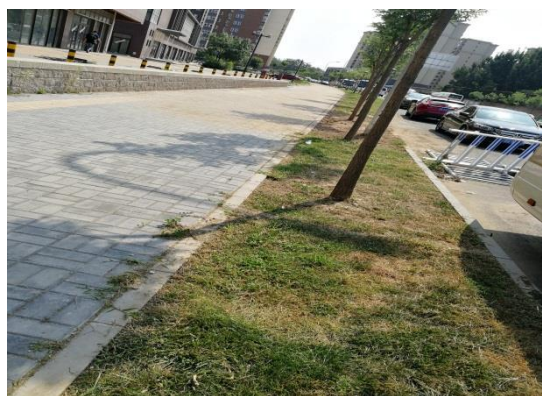
步道透水铺装及绿化带 (2020.6)
