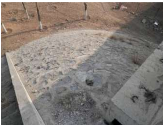
桥梁锥形护坡
